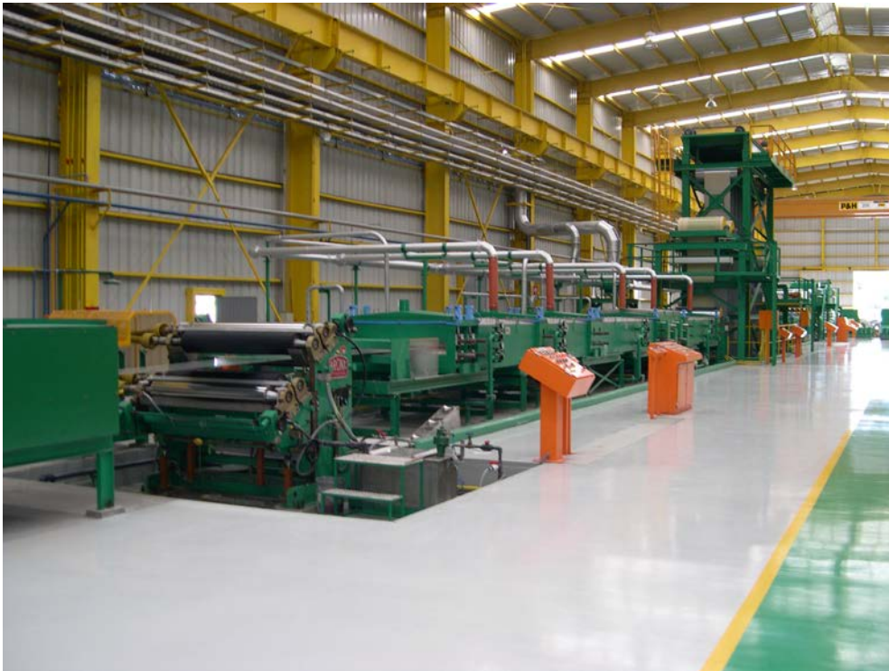
Typical cleaning and pre-treatment section of a coil paint line
