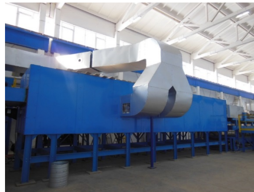
Figure 6.0: Gas Fired Convection Paint Curing Oven for 40 m/min Coating Line
